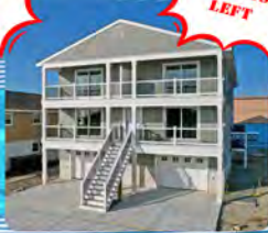
104 31st St S New Construction
