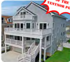
107 S Cambridge New Construction, Beach Block
