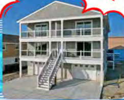
104 31st St S New Construction
