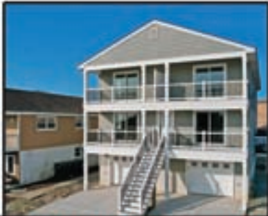
104 31st Street South • Brigantine 4 Units - New Construction
