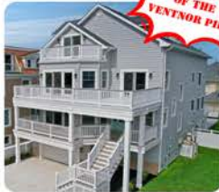
107 S Cambridge New Construction, Beach Block
