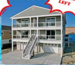
104 31st St S New Construction
