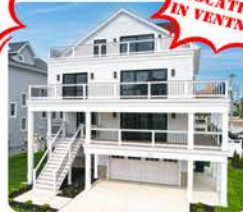
109 S Cambridge New Construction, Beach Block
